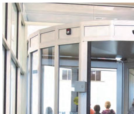
The revolving door's Segmented® drum design, unique to Horton, allows for smooth action while eliminating the need for costly curved glass.
