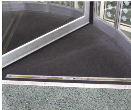
The door's object detection technology (in floor and overhead) senses undesirable and dangerous objects and prevents reentry, shutting the door down and sounding an alarm if something is detected.
