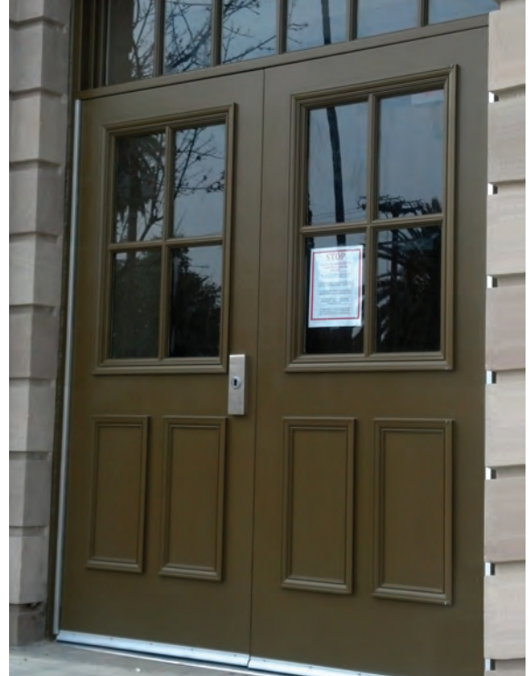
Primary Gathering Building with Krieger blast resistant door up to 1.0 PSI LLOP
